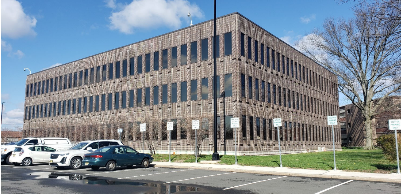
Overview of F&A Building From the Northeast
