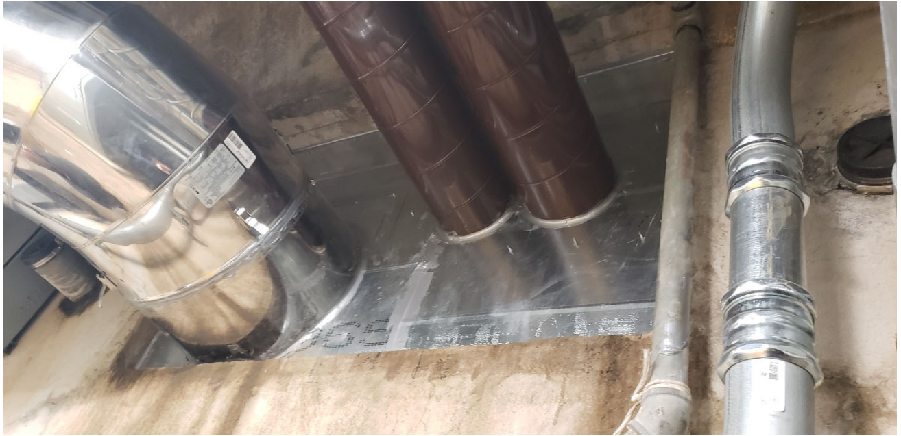
Intake/Exhaust Vents at Area South Facade - Interior
