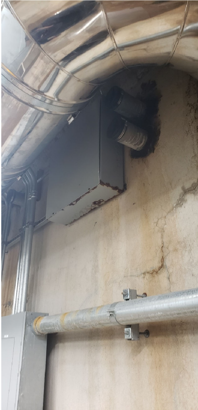
Capped Penetrants at South Wall
