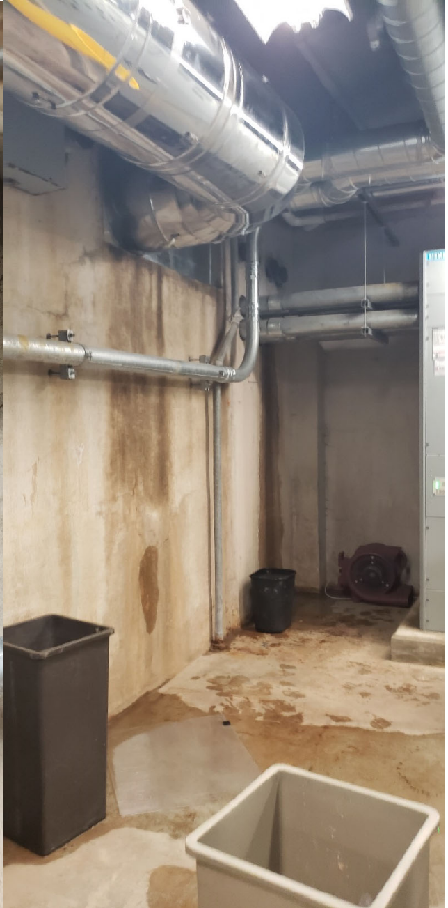
Southwest Corner at Electrical Room
