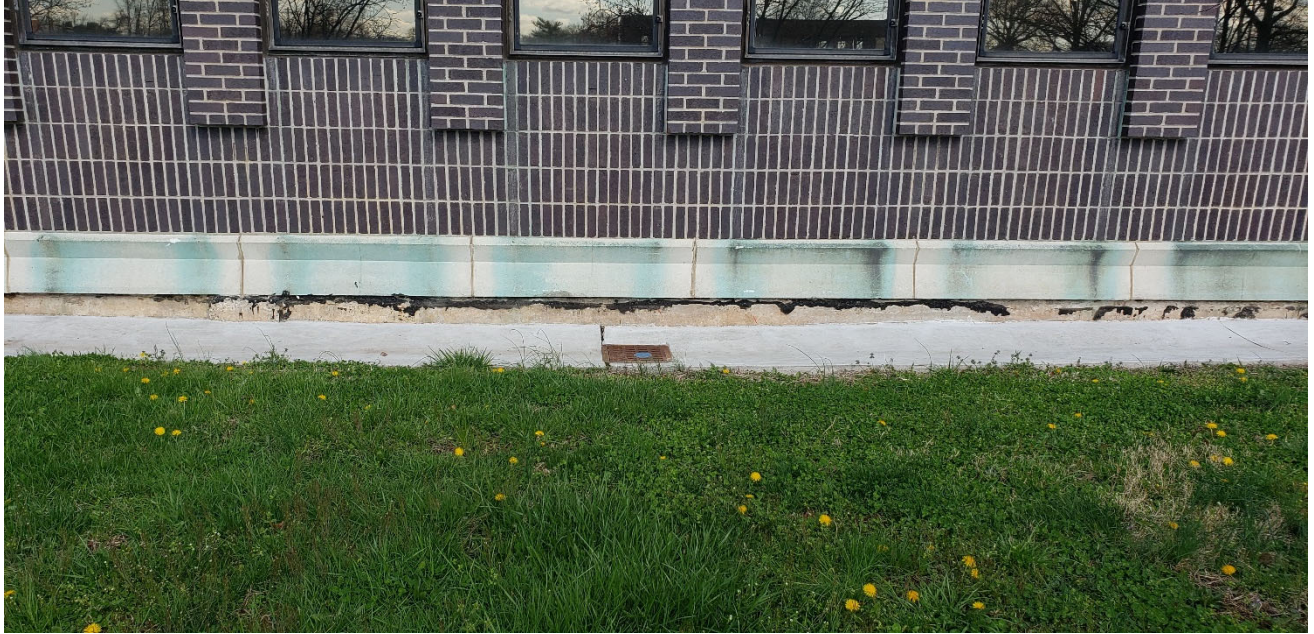
Base of East Facade
