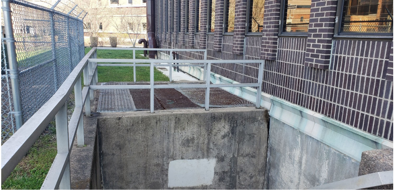
Existing Stair and Ramp Construction at South Facade
