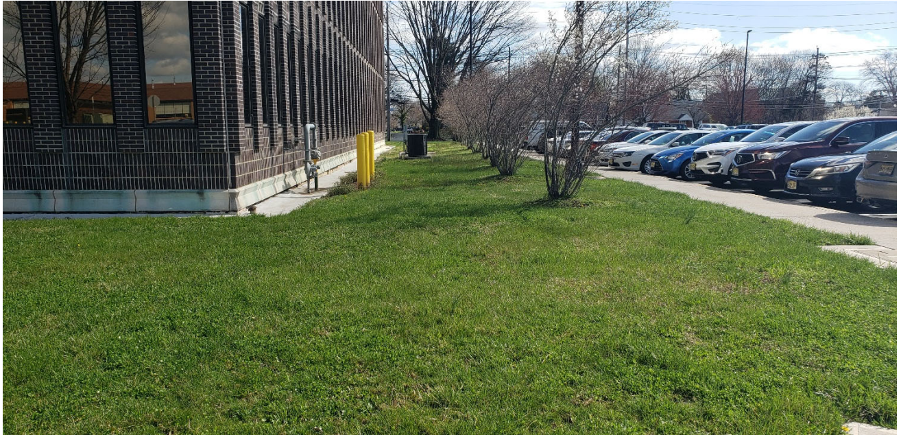
View of Grade Along East Facade Looking North
