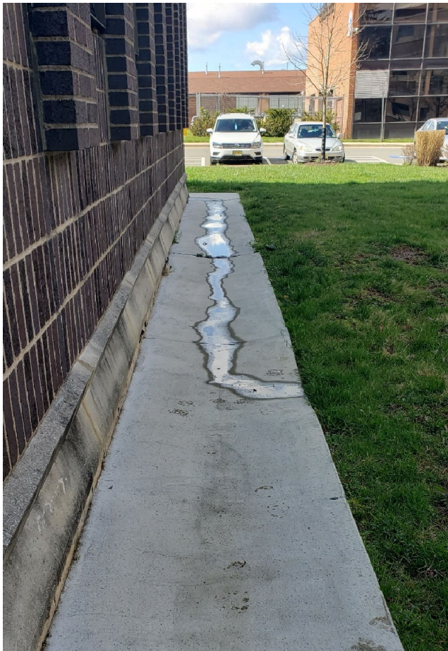
Concrete Apron at West Facade
