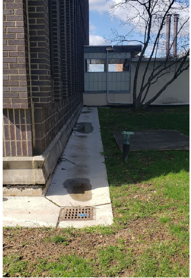
West Facade Looking South
