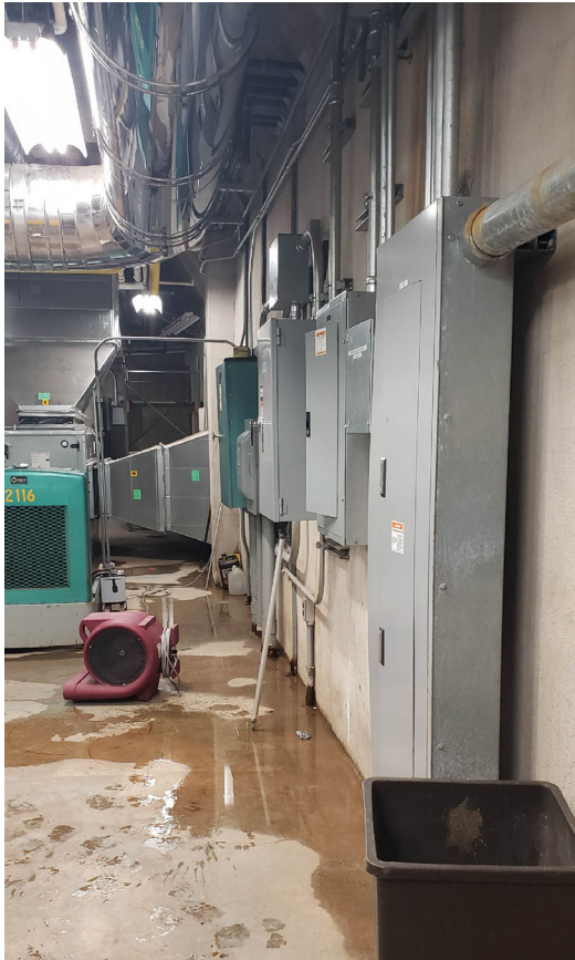
South Wall of Electrical/Mechanical Room
