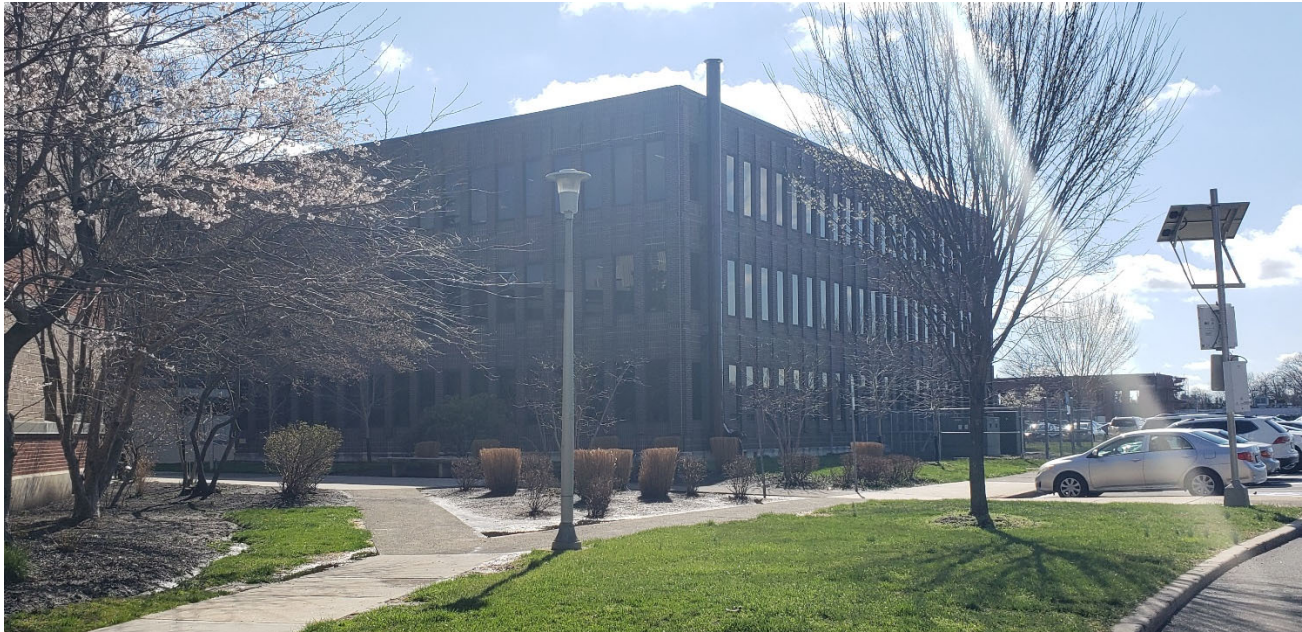
Overview of F&A Building From the Southwest
